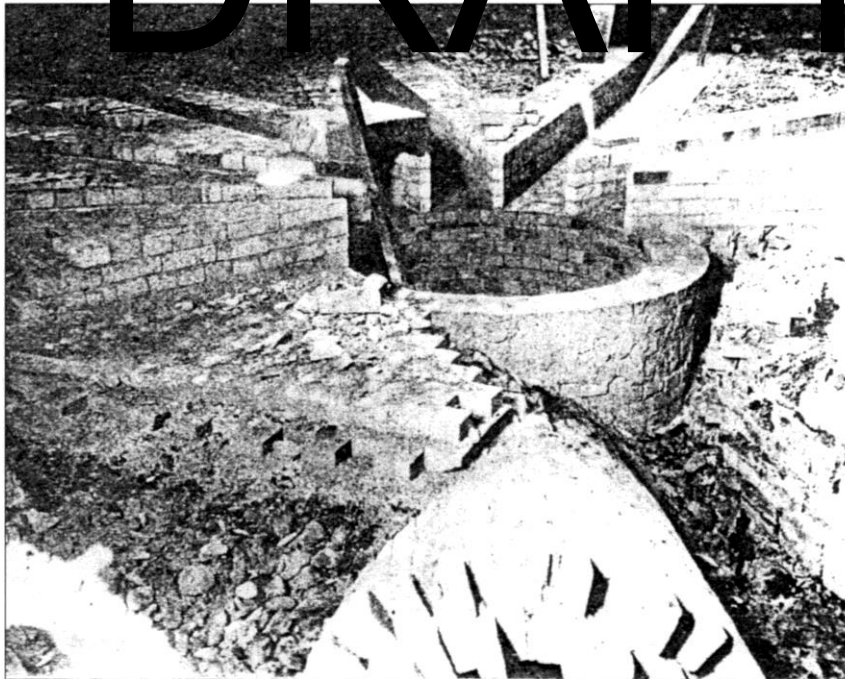
Floor of a Carnegie brick kiln. From California Division of Mines and Geology.
