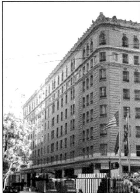
Sheraton Palace Hotel in San Francisco is faced with Carnegie brick and terra cotta. Dan Mosier Collection.
