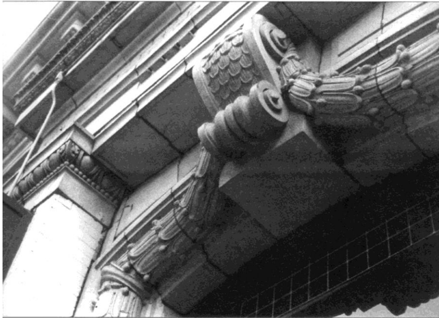
Carnegie terra cotta, Methodist Book Concern Building, San Francisco. Dan Mosier Collection.
